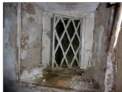
Photo 23 Cast-iron lattice window
