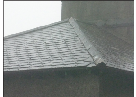
Photo 04. Missing slate to roofslope RS04
