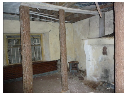
Photo 21. Tree trunks used to prop floor
