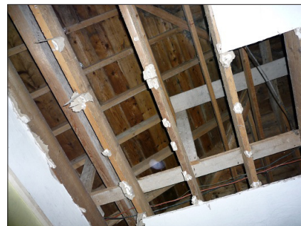
Photo 29. Collapsed ceiling
