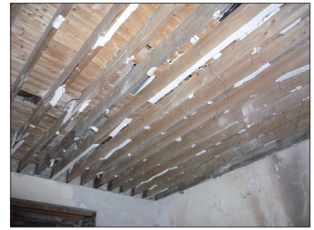
Photo 27. Collapsed ceiling plaster
