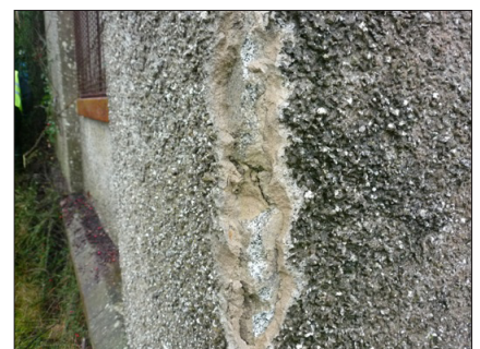
Photo 09. Underlying granite walling
