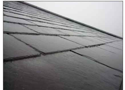
Photo 05. Slating in good condition
