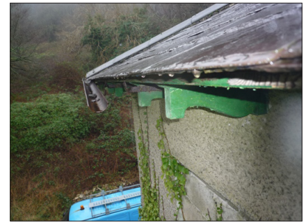
Photo 10. Missing section of gutter
