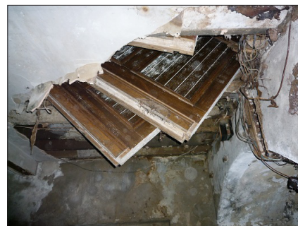
Photo 20. Collapsed ceiling room R001
