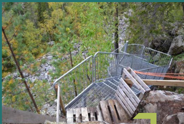
Figure 11: Top of the Galvanised Staircase constructed to guide walkers over heavy rock and scree deposits to the bridge.
