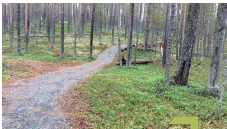
Figure 6: A ravel rail in Hossa National Park. Drainage is achieved through path sloping and 'rolling dips'
