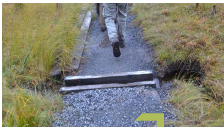
Figure 13: Experimental path through floating mire with timber water bar and edging
