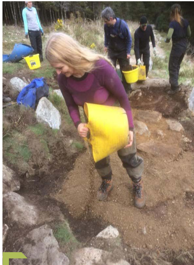
Natural aggregate was extracted from pits and used to create a firm path surface on the Glen River path at Slieve Donard. To the rear, stone steps were realigned to improve the path line and account for changing gradients
